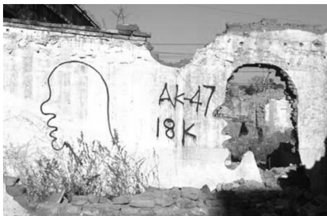
Figure 2 Demolition, Forbidden City, Beijing 1998
